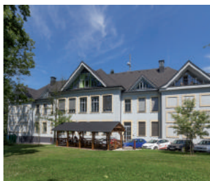
NAM system headquarters
